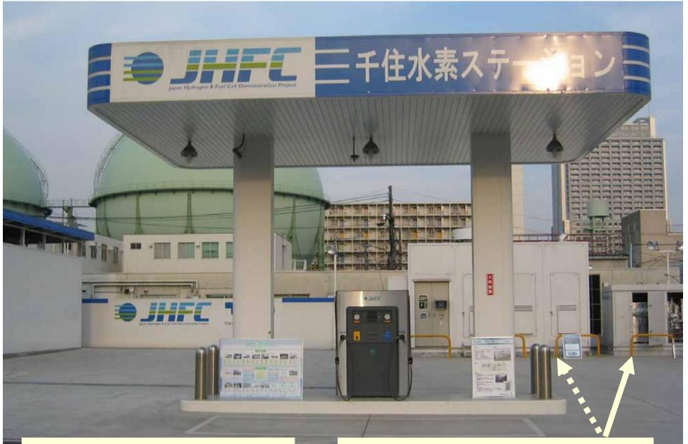
Hydrogen Station Operating in Senju Tokyo Membrane Reformer by Tokyo Gas Co. Volume=1/3 Space=1/2 as Compared with the Conventional Reformer
