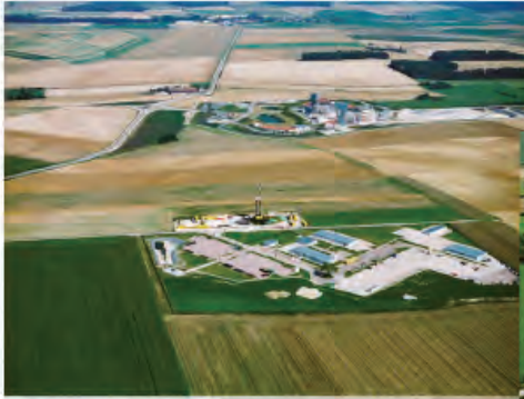
The development area in the forefront (Saudron area), a drilling platform with a operating rig and the URL in the back
