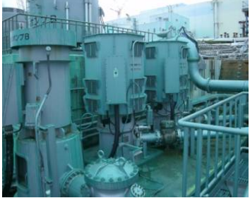
Unit1 PCV cooling sea water pump
