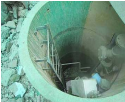
The pits filled with debris inside after the lid broke due to the tsunami
