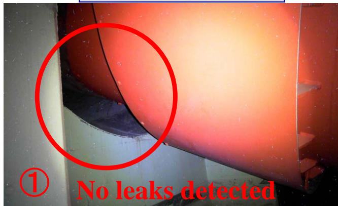
Vent pipe sleeve end
