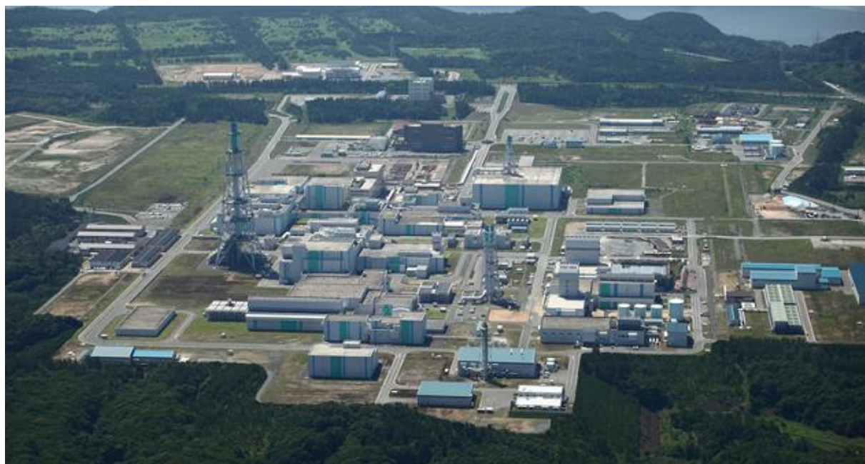
Rokkasho Reprocessing Plant ( http://www.jnfl.co.jp , as of January 27, 2016)
